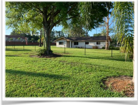
An early photo of SJCA fence installment.
